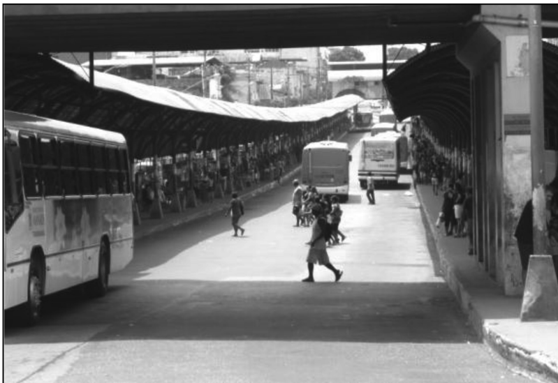
Figura 4 - Terminal 1 Constantino Nery: interior
