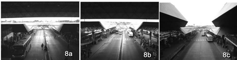
Figuraa 8a - (Terminal 3), 8b - (Terminal 4) e 8c - (Terminal 5): Interior
