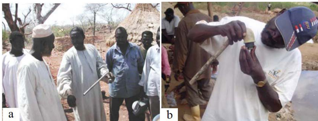
Figure 7. a) Building RHYM Retorts in Sudan and b) Munhena, Mozambique.
